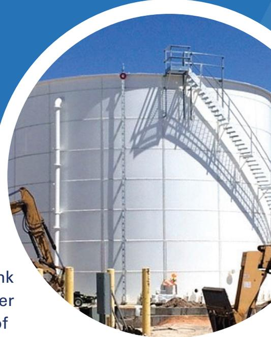
AST Storage is a tank manufacturing leader and the developer of DuraCoat, an epoxy powder coating system that sets an industry benchmark standard for its exceptional durability at an economical price. The first tanks with DuraCoat were produced in 2003, and nearly 20 years later the finish is still performing like new – creating cost savings and easier maintenance for owners everywhere.
